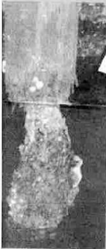
Damaged Piling
