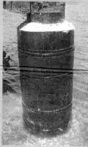
Severe Damage Piling Encapsulation
